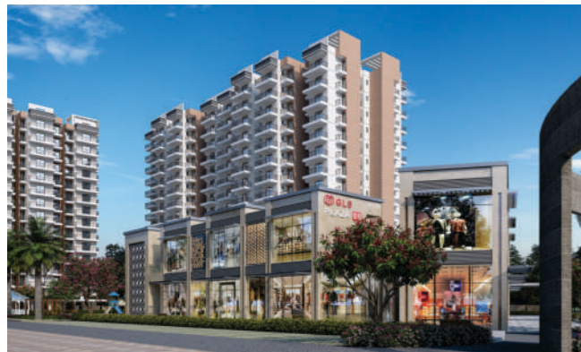
AVENUE 86 | Construction ahead of schedule
