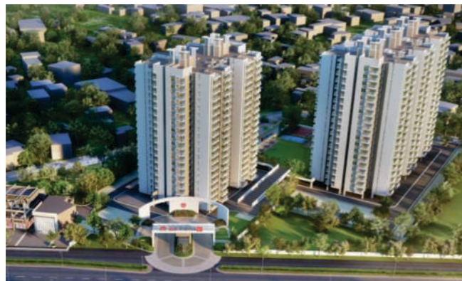
AVENUE 81 | Construction ahead of schedule
