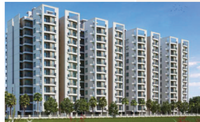
SOUTH AVENUE | Construction ahead of schedule
