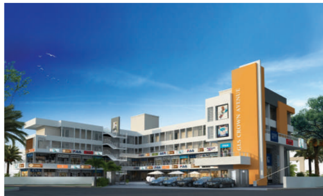
CROWN AVENUE | Construction ahead of schedule
